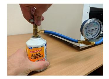
Step 11) Check the pressure on the gauge at equilibrium.
