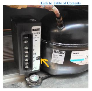
Step 6) Separate ECU from compressor. Take off screw side first.
