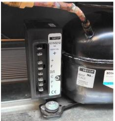
Step 12) Reconnect wires to ECU. Make sure they are the same as before based on picture taken. Example wiring diagram is also below.
